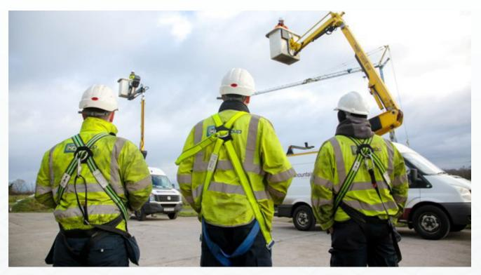
**Platform Positioning:** Position the platform within the guidelines set from the working envelope by this it allows the workers to reach the work area and minimise risk of overreaching or having the need to climb out of the platform.
